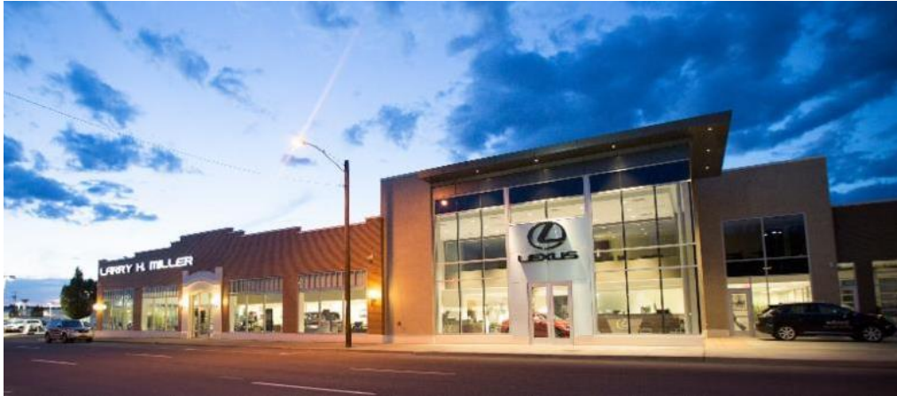
Washington State Energy Code (WSEC) 2012 air barrier "building test" services were fulfilled for the new addition of Lexus of Spokane.
